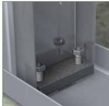
Install nuts/washers on anchors.
