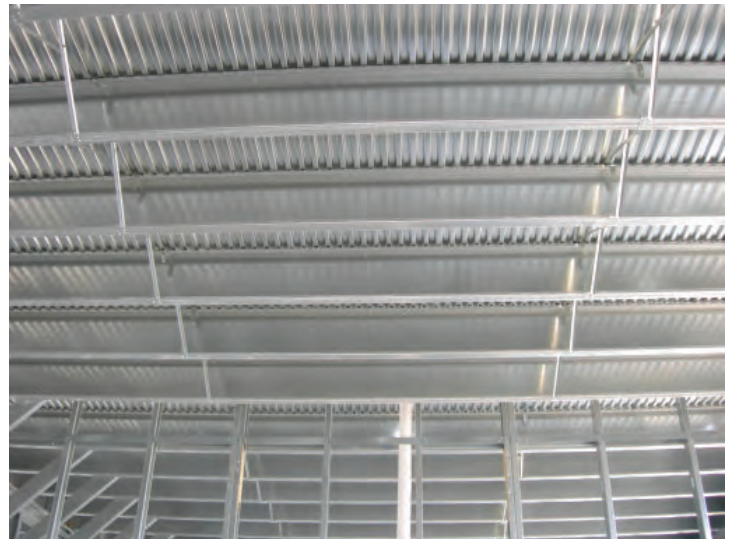
Cold-Formed Steel Joist
