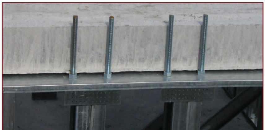
Fig. 2: Sheathing should not be attached directly to the StiffWall Column. Attach the sheathing to the adjacent studs.
