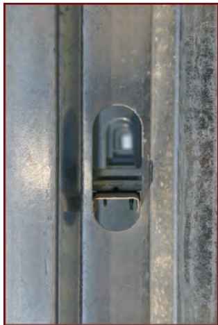
SigmaStud's punchouts provide a convenient avenue for electrical chase.
