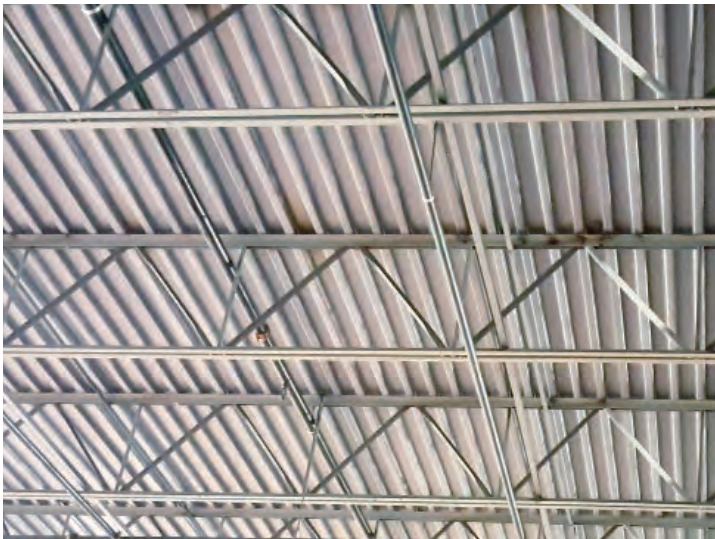
Composite Bar Joist
