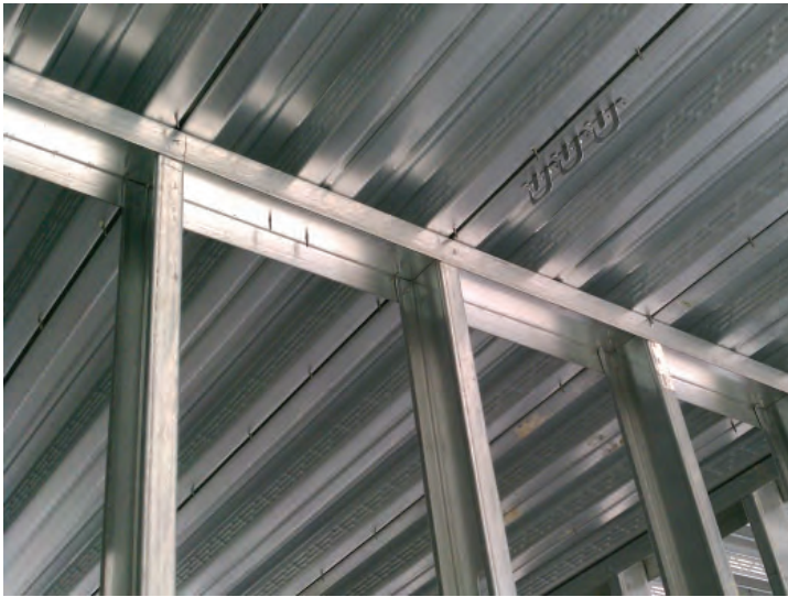
Composite Steel Deck
