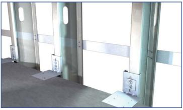
VertiClip SLF used with one flat strap bracing on the outer flange of studs to resist torsional effects.
