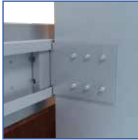
6 Hole Fastener Pattern
