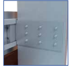
9 Hole Fastener Pattern
