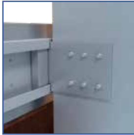
6 Hole Fastener Pattern
