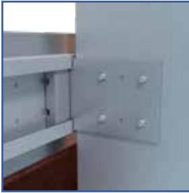
4 Hole Fastener Pattern
