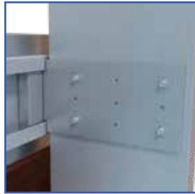
4 Hole Fastener Pattern
