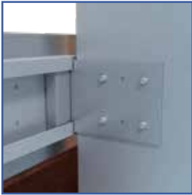
4 Hole Fastener Pattern
