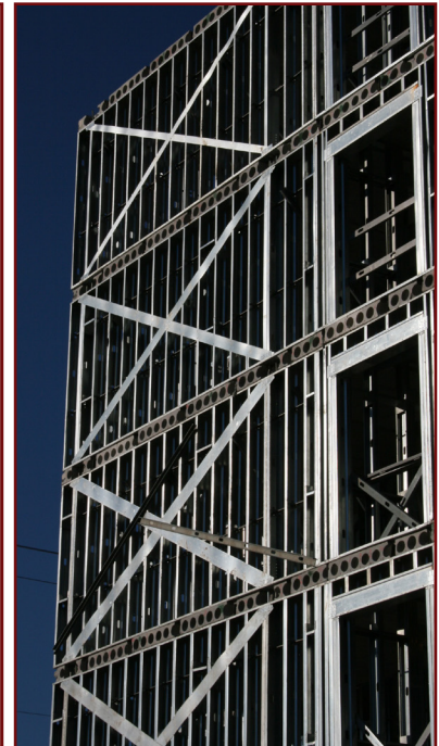
Fig. 3: Shear walls should be stacked vertically.
