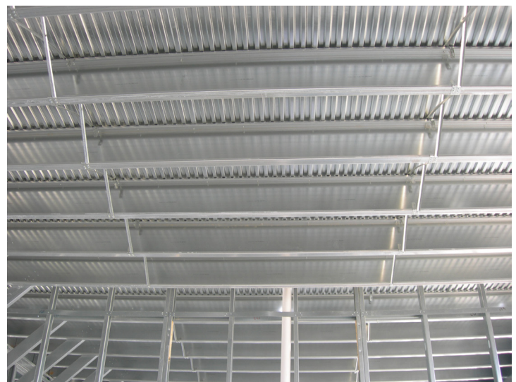
Cold-Formed Steel Joist
