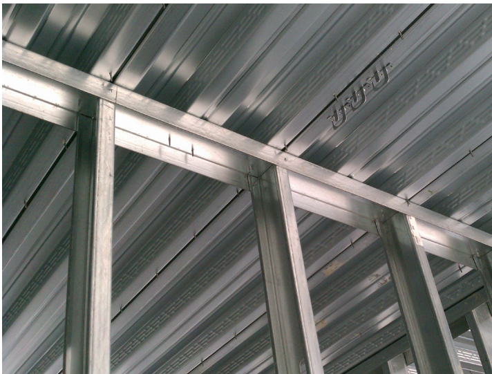
Composite Steel Deck
